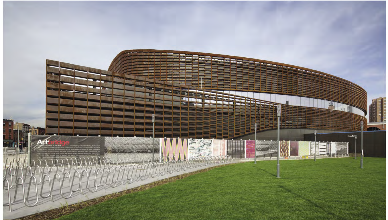
Above Internal truck elevators and turntables eliminated the need for ramps to loading docks, allowing the arena to have more of a storefront presence in downtown Brooklyn.
