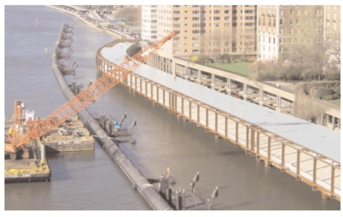
Engineers attached steel pipes measuring 11 feet in diameter to the roadway's waterside edge to act as a "fender" for errant ships.
