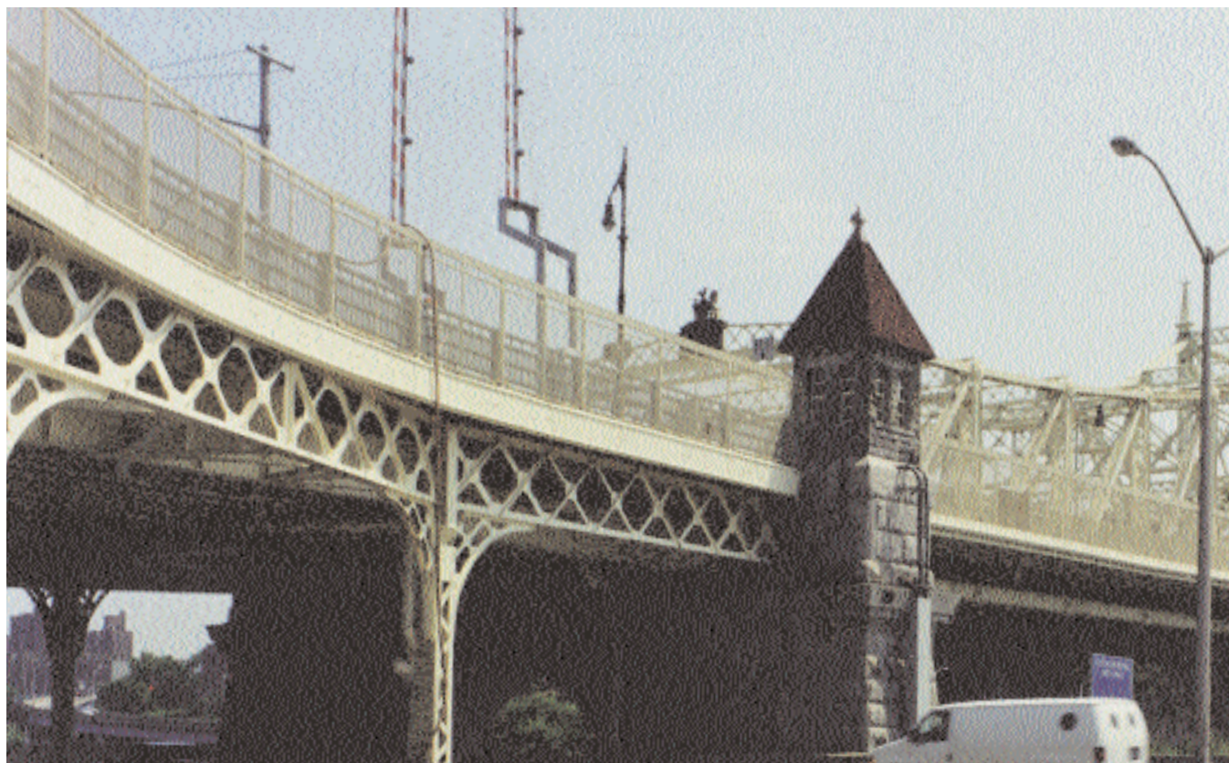
The roadway decks were replaced in their entirety while maintaining traffic in both directions and the work could only be done during Yankee off-seasons.
