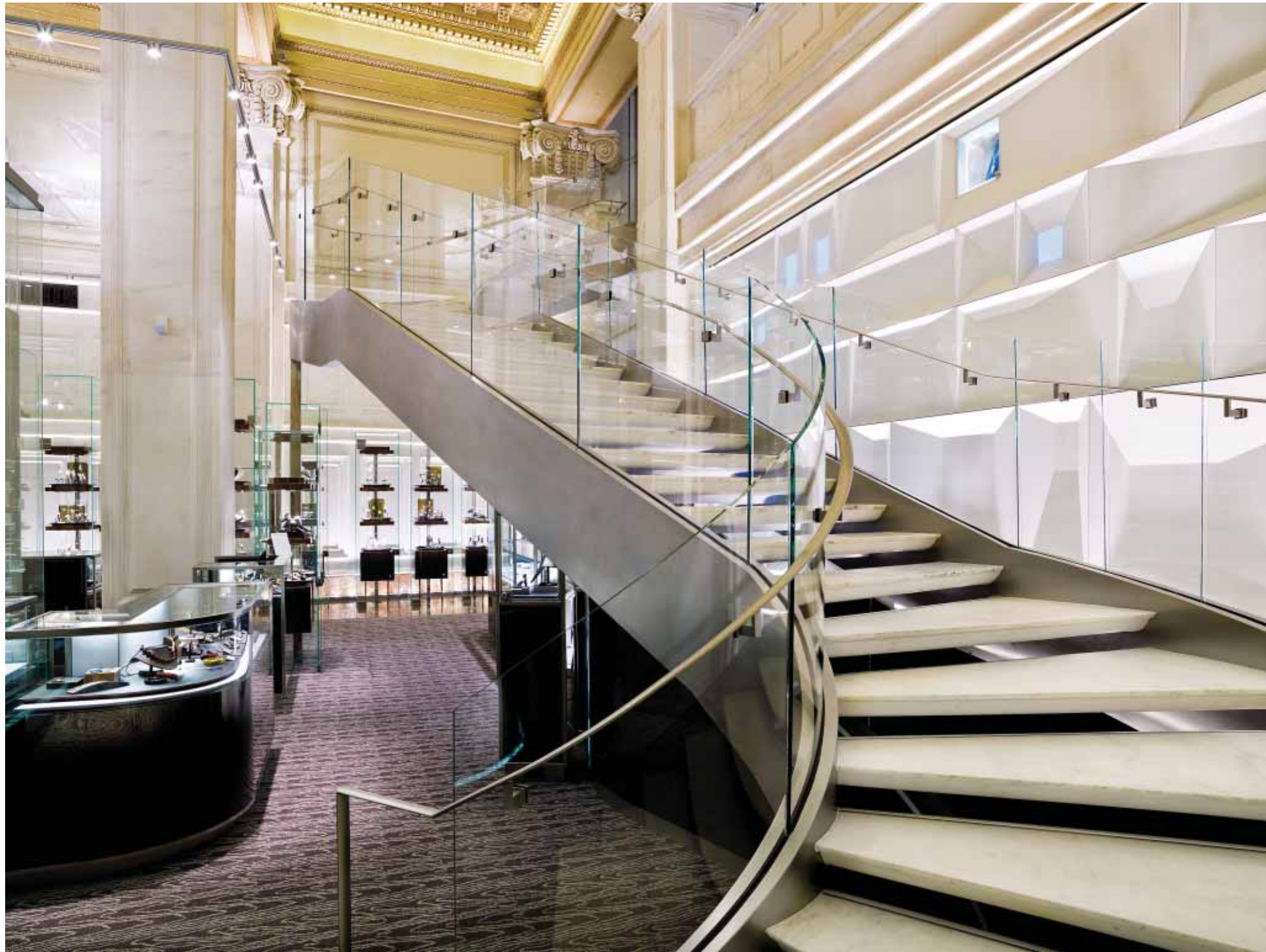
Above The S-shaped stair with its Starphire glass railings was tirelessly soldered and finished to achieve a seamless look. Right The existing facade.
