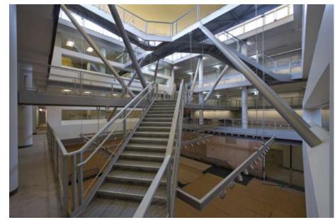
Facing page Bridge sections were site-welded to each other in mid-air, then connected to the concrete slab floor, stairways, and other reinforcements.
