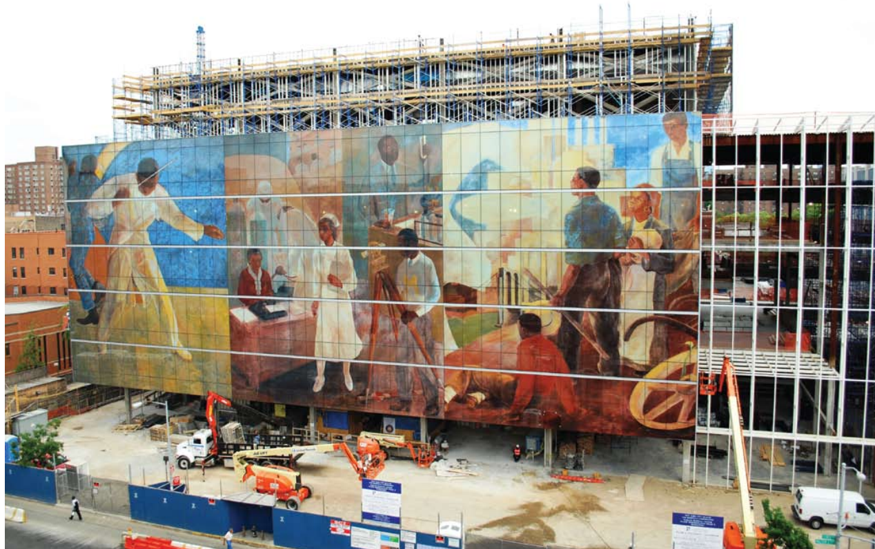
Above Vertis Hayes's Pursuit of Happiness is digitally printed on the building's six-story glass facade mounted on a concealed steel structure.
