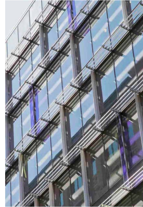
Above The curtain wall's glazing includes low-iron glass, clear vision glass, clear vision glass with frit on the No. 2 surface, and fritted laminated spandrel glass. It is accented by vertical anodized aluminum fins and by vertical blue and yellow dichroic glass fins.
