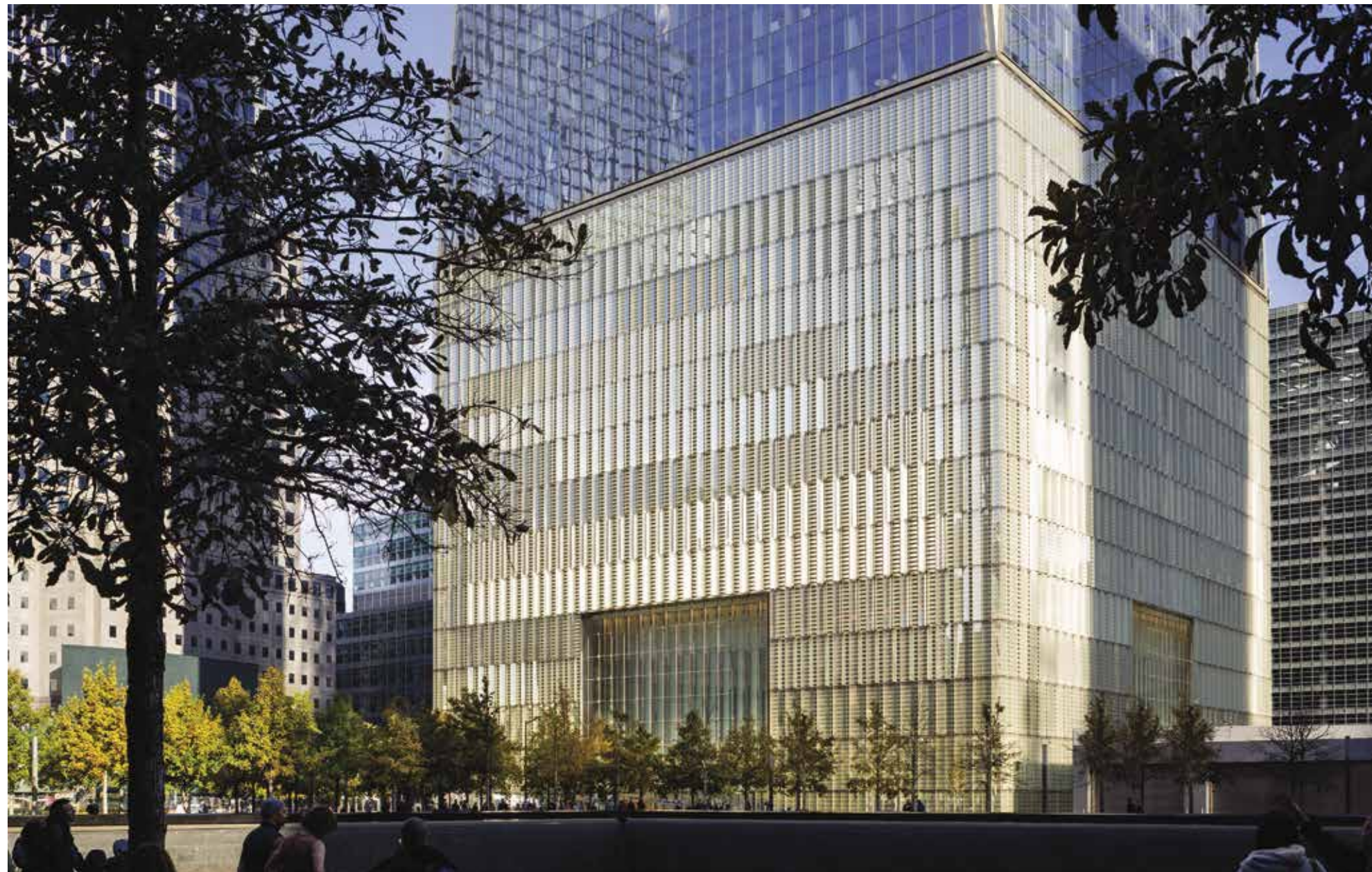
Above More than 4,000 laminated glass fins and stainless steel slats form the face of the podium, accommodating mechanical ventilation and breaking down the mass of the building's base.
