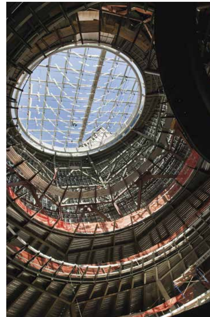
Above left Within the pavilion, the outer branches of V columns support the pavilion roof, while the inner branches support the oculus and frame the center's dome. Above right A circulating stair connects the center's shopping and dining venues.
