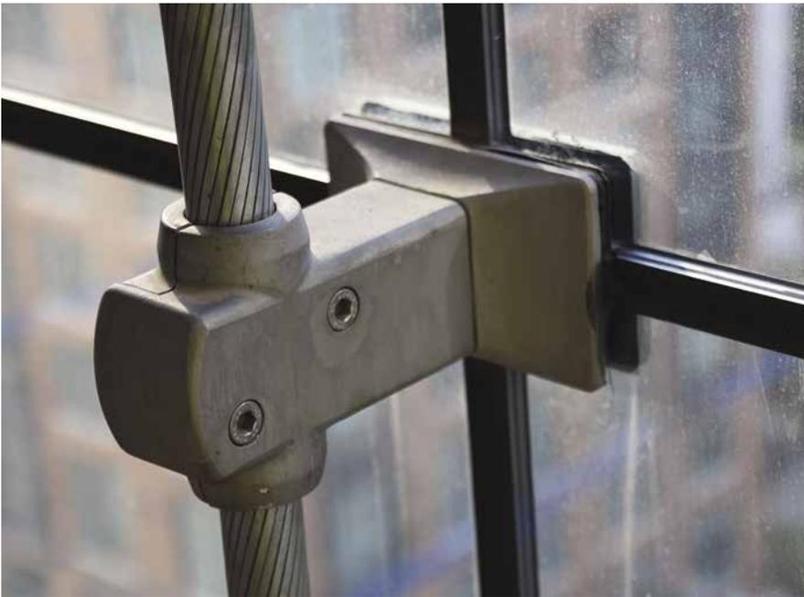
**Top** A stainless steel cast patch fittings on which cable wall glass is set. The fitting connects to a Galvan link locked tension cable—with such a large glass load, stainless steel cable was not an option due to limitations in stainless cable diameter and strength.
