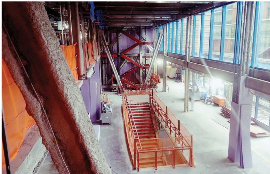
Clockwise from top Milstein's double-height library is framed by U-braces and anchored by a cantilevered, switch-back feature stair. The stiffness achieved by using braced frames, expressed on the ground floor of the library, allowed for an overall more efficient structural frame and supported Milstein's height. The steel structure of the U-braces and stair visible during construction.
