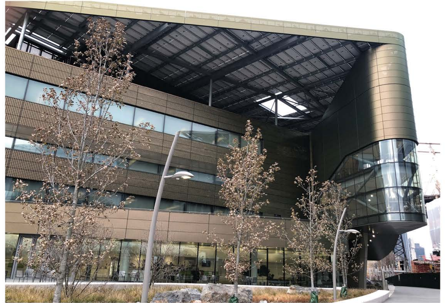
The feature stair cantilevers over the pedestrian path between Bloomberg Center and the neighboring Tata Innovation Center.
