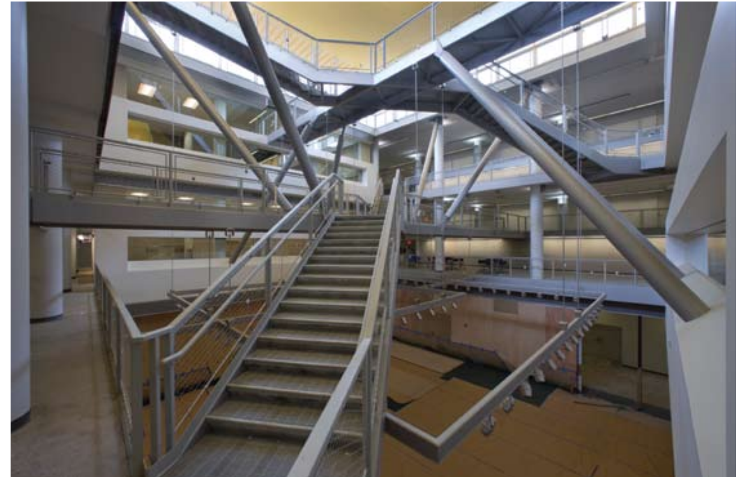
Facing page Bridge sections were site-welded to each other in mid-air, then connected to the concrete slab floor, stairways, and other reinforcements.
